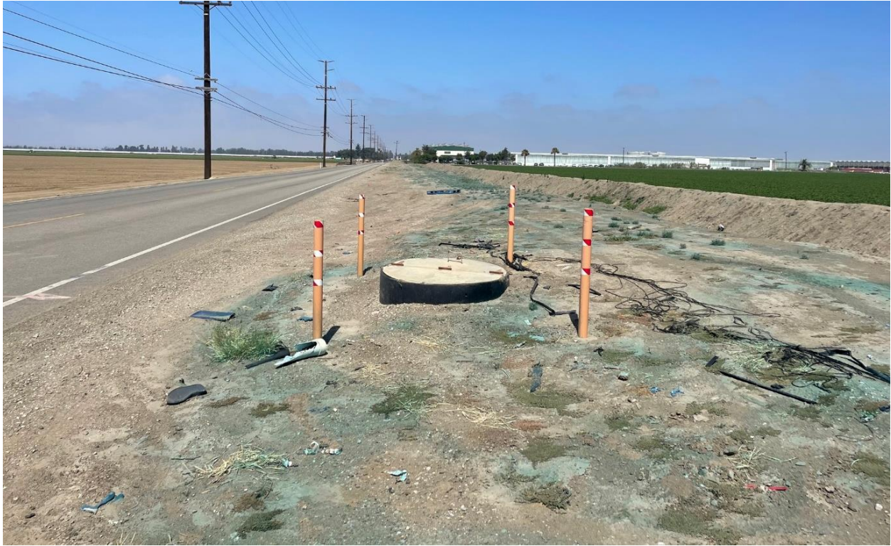
Figure 7 Underground Utility Within Project Site, Facing West
