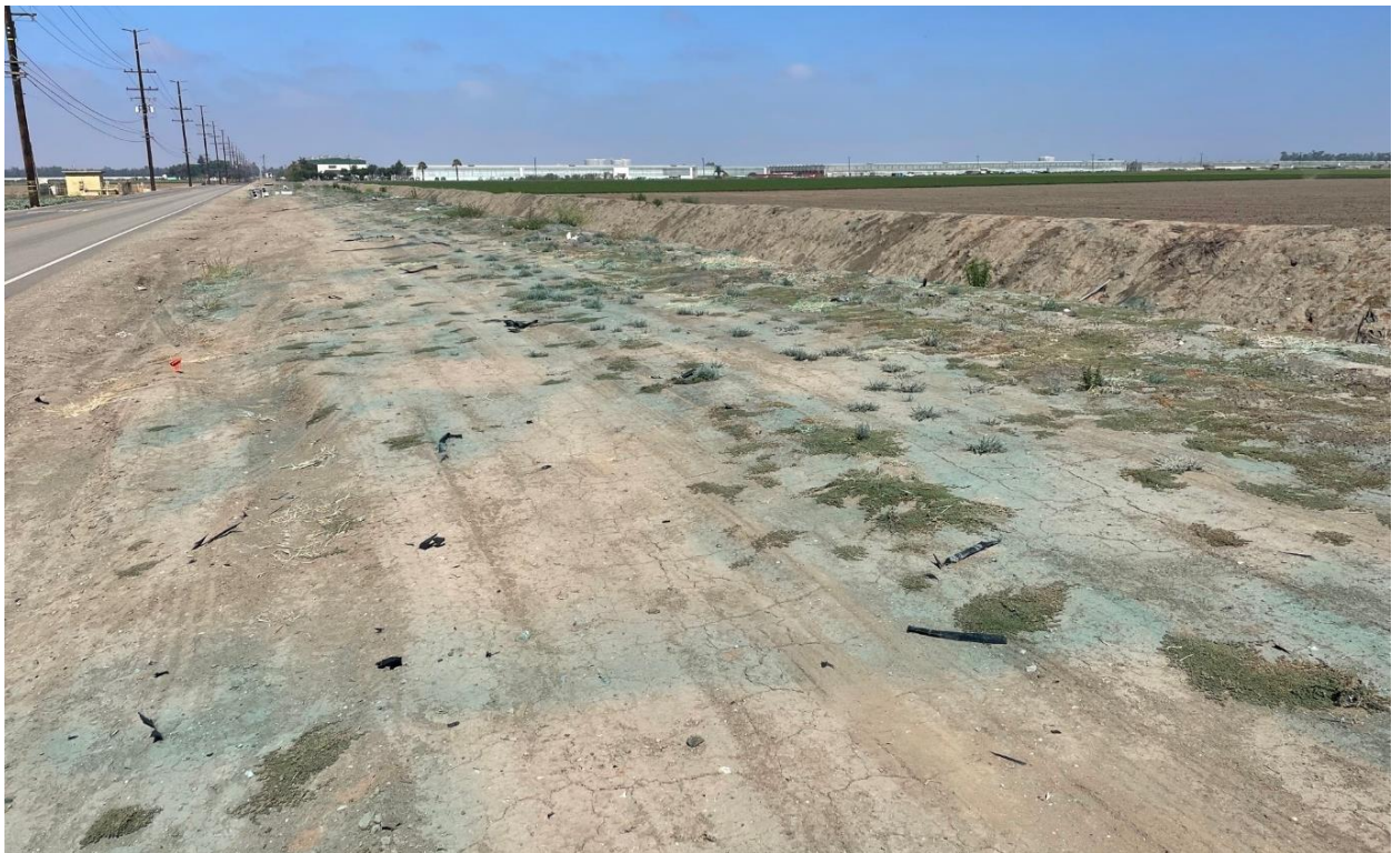
Figure 6 Soil Discoloration, Facing West
