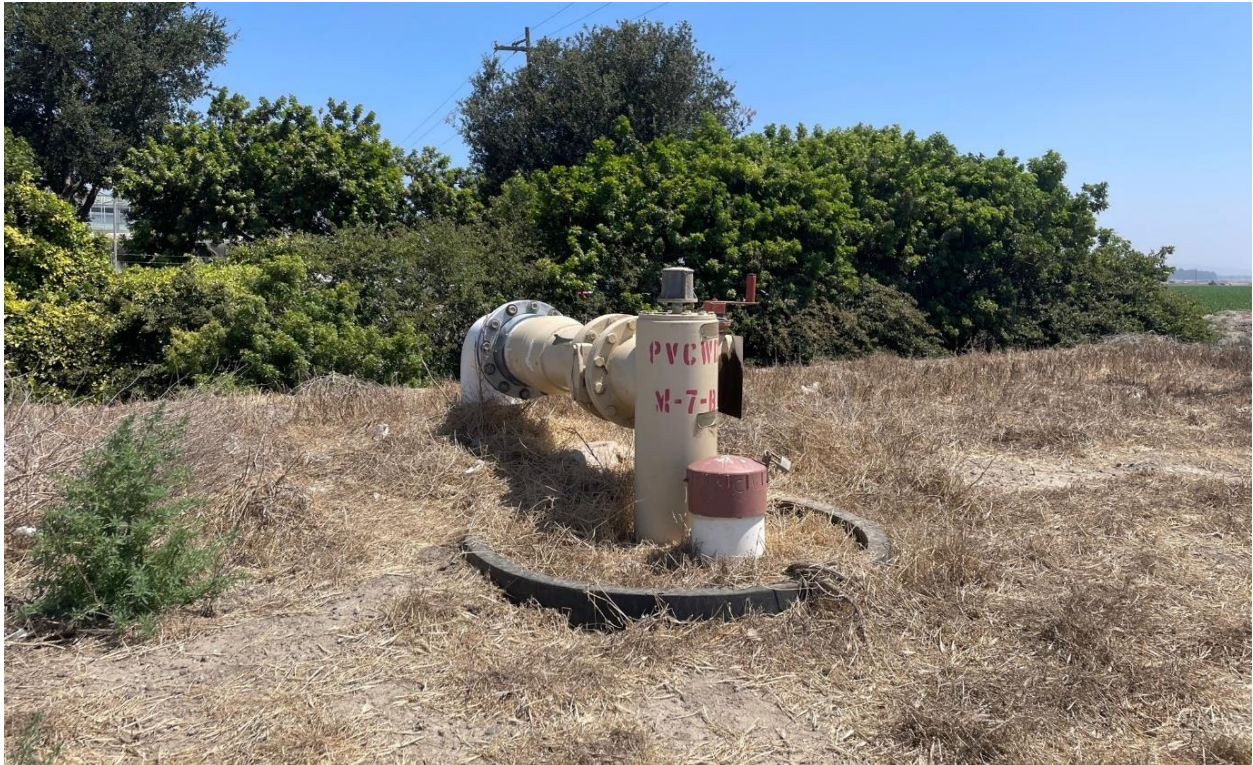
Figure 8 Underground Utility Within Project Site, Facing North
