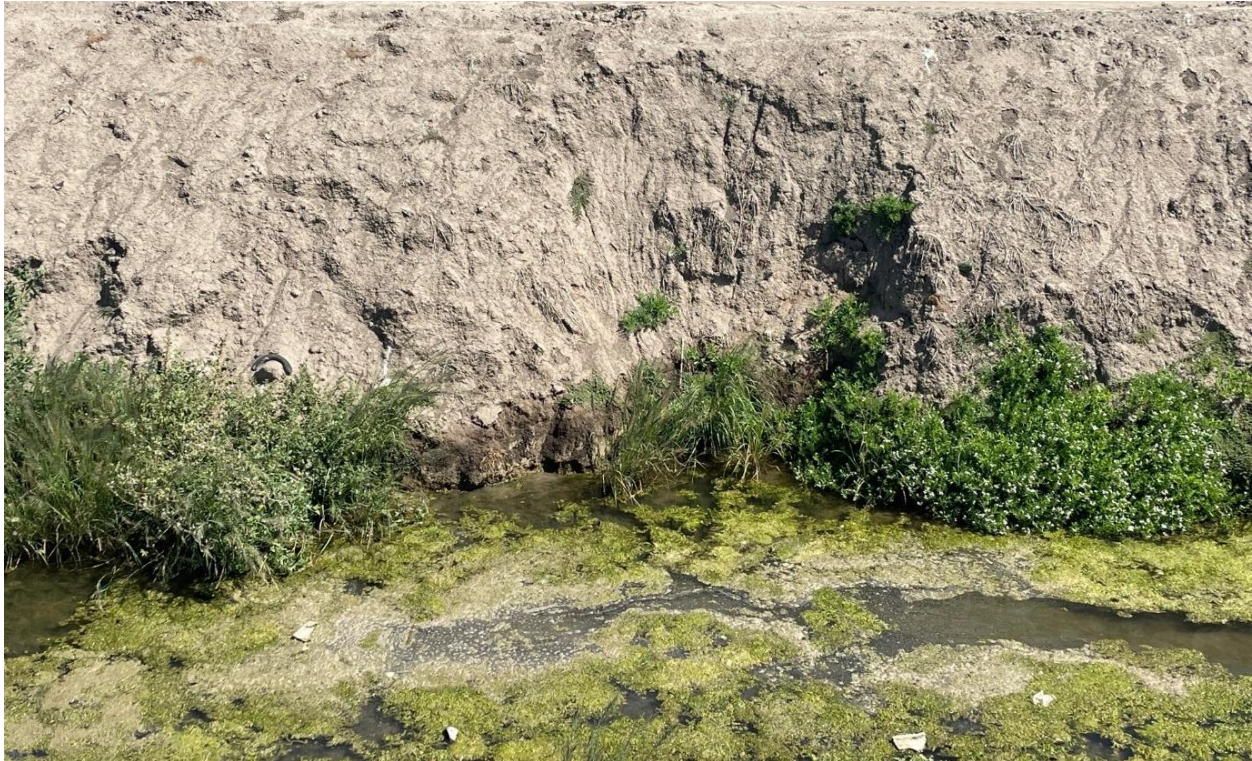
Figure 14 V-ditch Profile, Facing North
