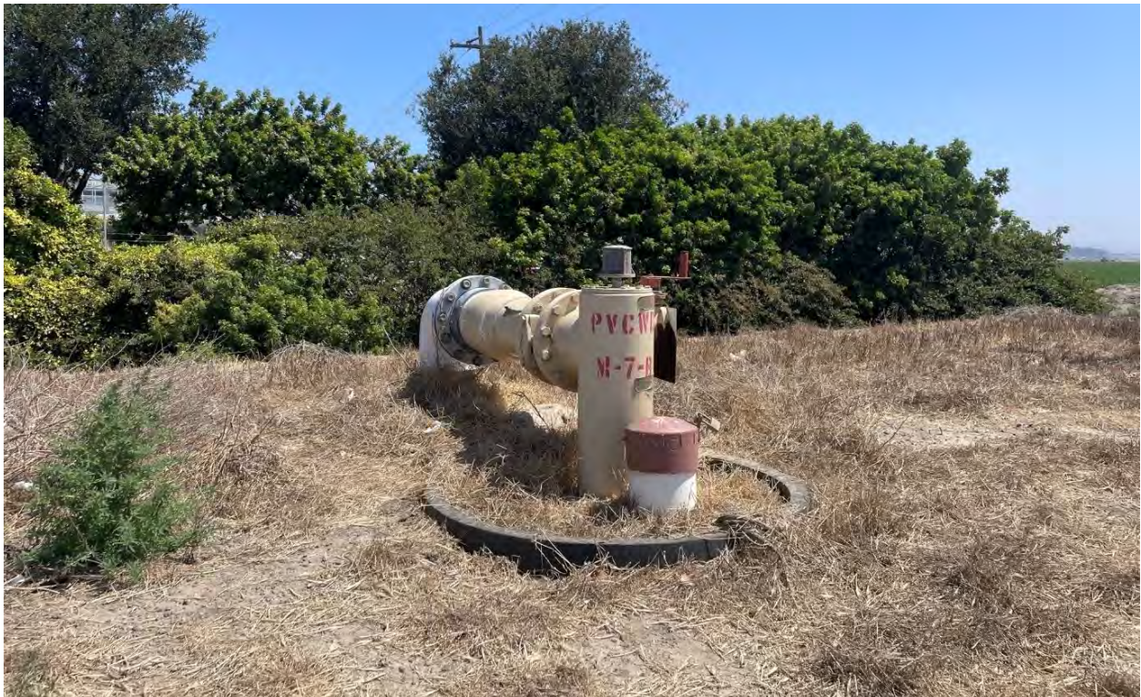
Figure 8 Underground Utility Within Project Site, Facing North
