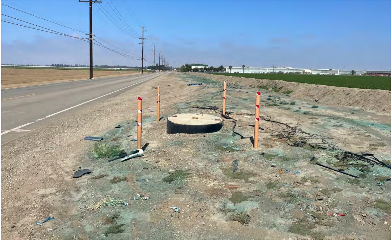
Figure 7 Underground Utility Within Project Site, Facing West
