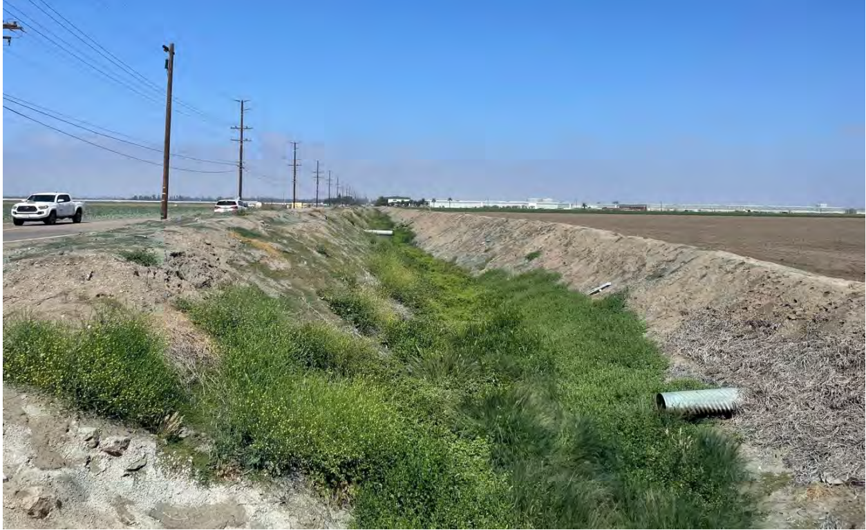
Figure 13 V-ditch Overview, Facing West
