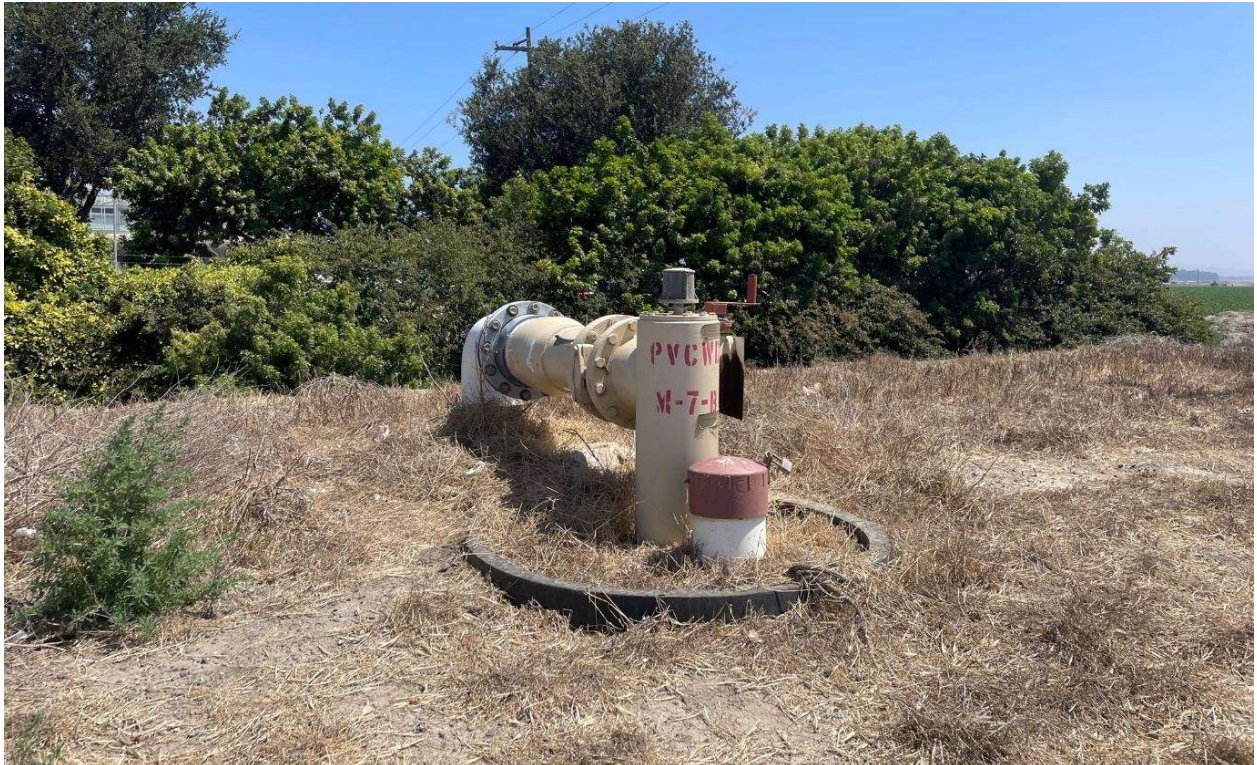
Figure 8 Underground Utility Within Project Site, Facing North
