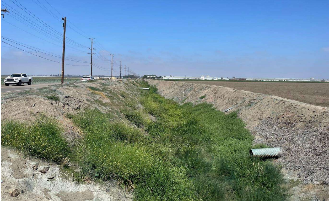
Figure 13 V-ditch Overview, Facing West
