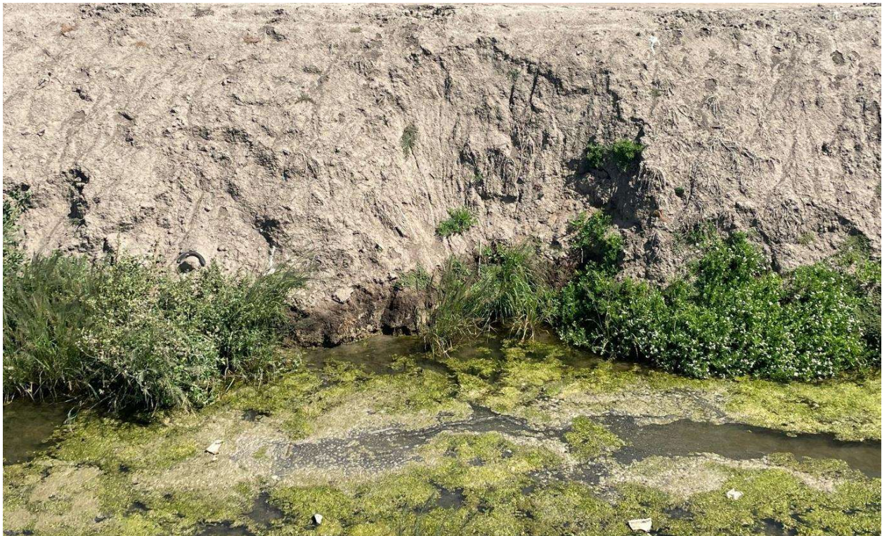
Figure 14 V-ditch Profile, Facing North
