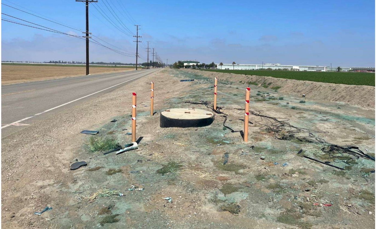
Figure 7 Underground Utility Within Project Site, Facing West
